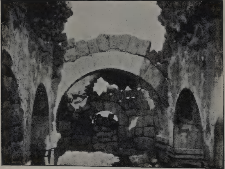
FIG. 106.—No. 16, interior of apse.
